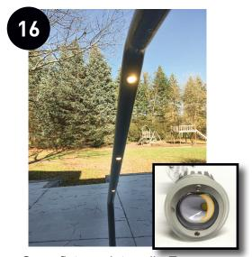
Snap fixtures into rail. Ensure direction of asymmetry is aimed in proper direction (half-moon on face of fixture shown in yellow in photo inset above). Seat gasket with finger to complete installation.
