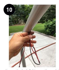
It may be helpful to gently assist the wire from the next hole down, but do not pull the wire tight within the rail. You'll need a small amount of extra wire after completion.
